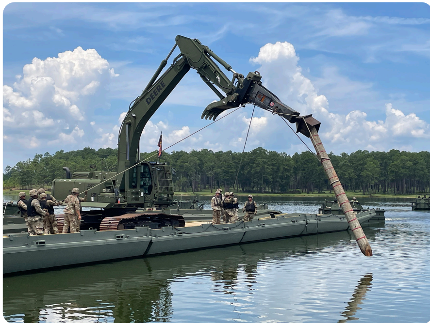
The 554th ECC and the 497th MRBC move a timber pile into place to test pile driving from an IRB.
