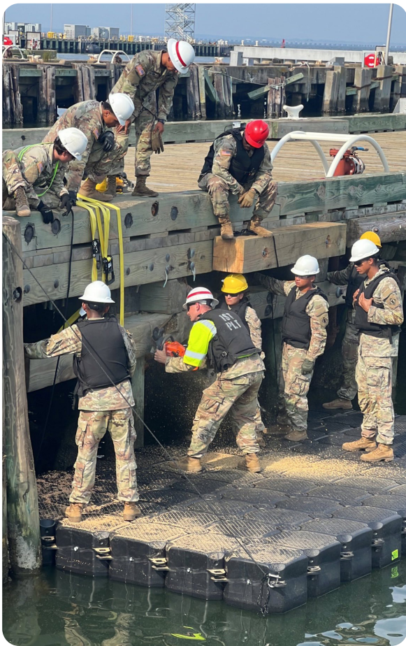
Soldiers deconstruct damaged sections of a pier.
