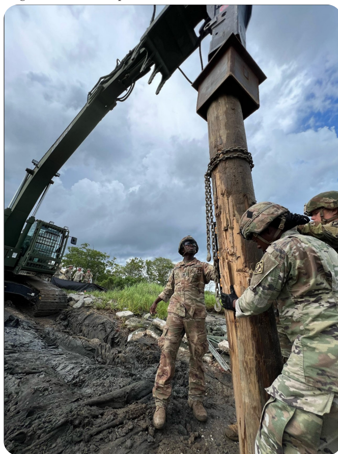
Soldiers drive a timber pile into place in the Savannah River during low tide.
