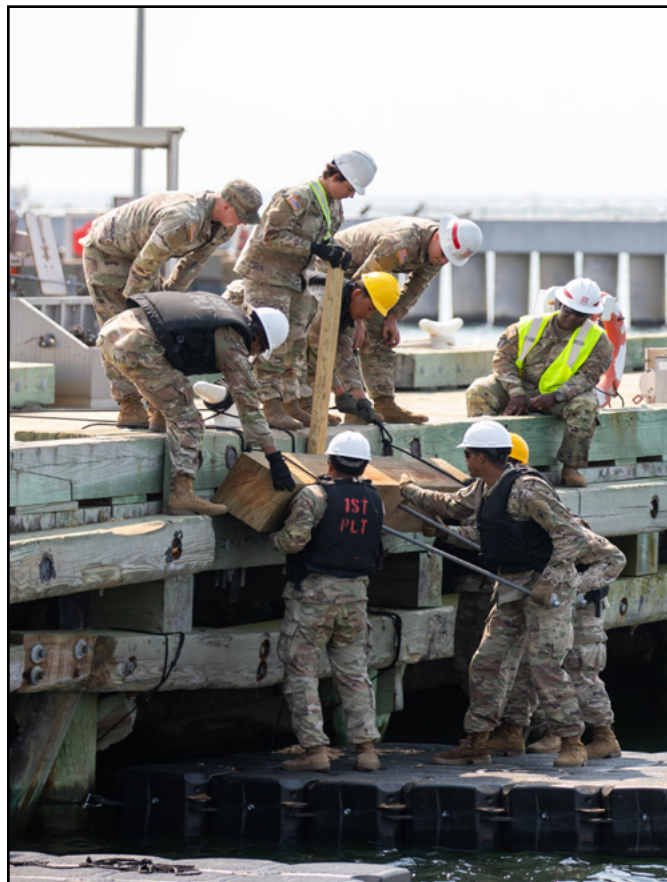
Soldiers perform carpentry work on a timber chalk.
