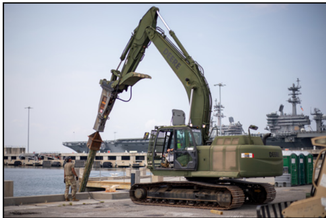
A Soldier uses a HYEX to drive a timber pile at Naval Station Norfolk.
