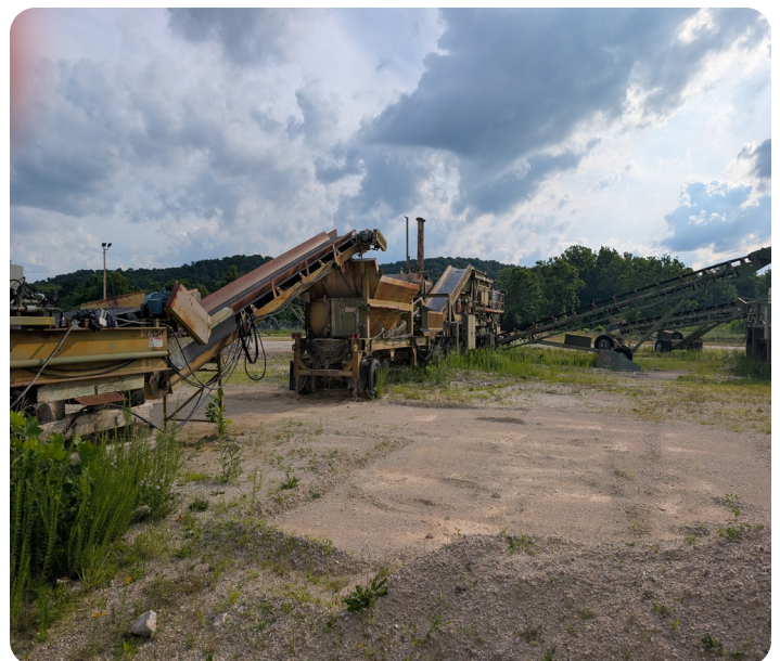
This the equipment is used for quarry AIT and is called the “crusher”
