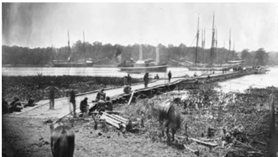
With boats in the water (center right) not attached to the main structure and soldiers clearly working atop the span, this photograph may show engineers constructing the pontoon crossing over the James River for Grant's move against Petersburg in June 1864.
