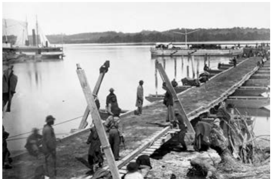
A pontoon bridge under construction at Belle Plain Landing, Virginia Library of Congress
