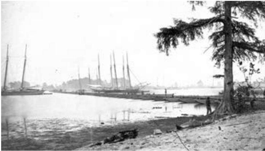
The completed bridge over the James in the late summer of 1864. This photograph also shows the heavy vessels used to stabilize it against the river's strong current and tidal changes.
