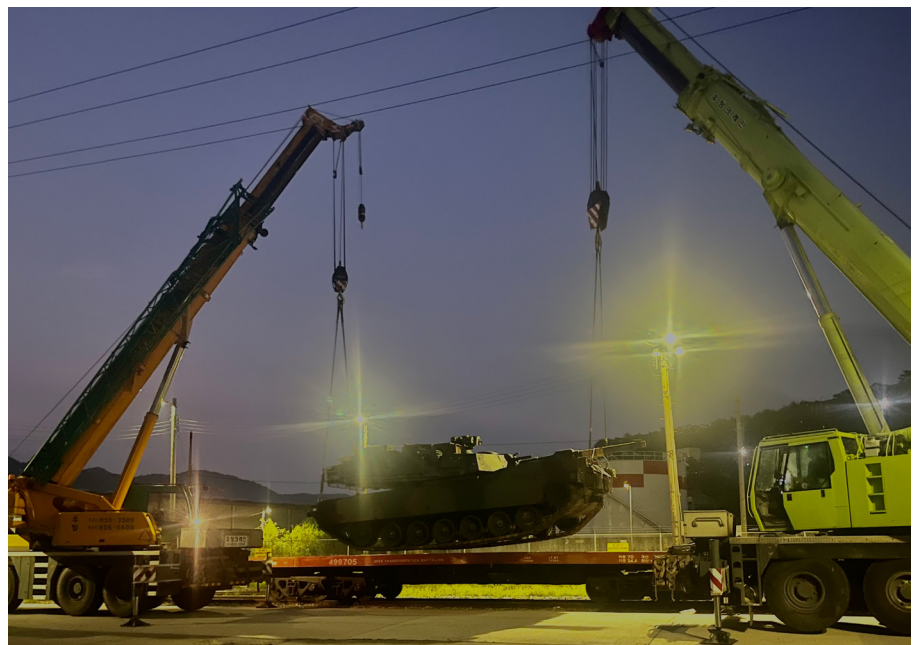
Figure 1. Cranes provide support to unload tanks at the Camp Casey Railyard, August 2023 (U.S. Army photo by MAJ Devin R. Osburn, Operations Officer, 3-61 Cavalry, 2nd SBCT, 4th ID)
