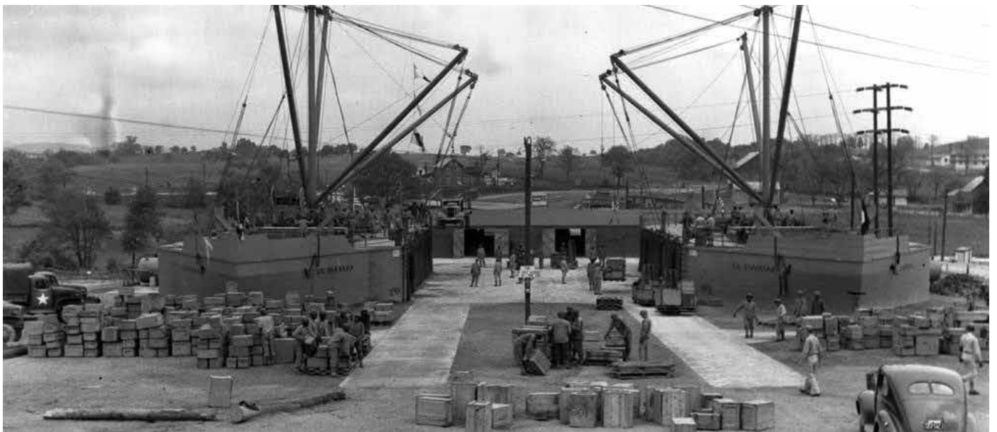
The mock wharf with “land ships” used for training stevedores at Fort Indiantown Gap.
